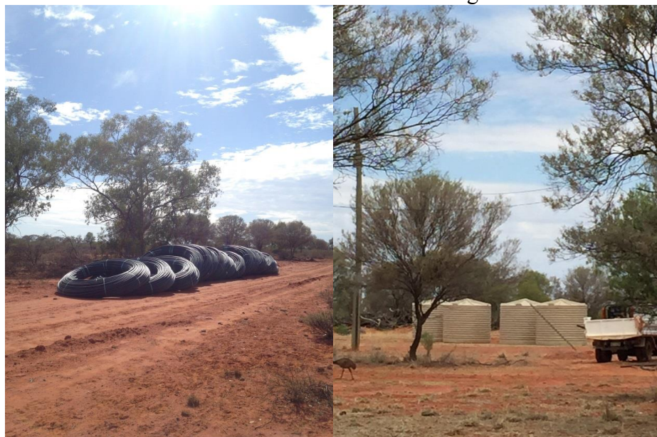
Photo 2 and 3: Materials on site and waiting installation.
