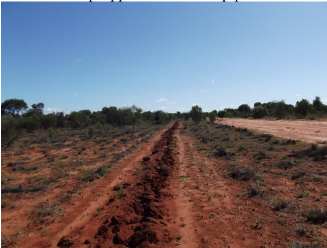
Photo 1 : Deep ripped channel for pipe
