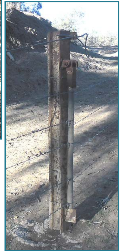
Left: The flood fence anchor point.
